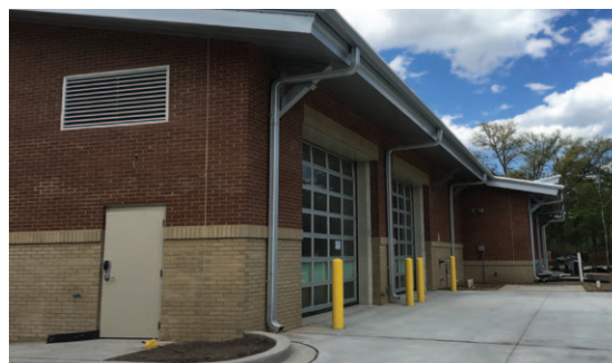
Fire stations such as Station 6 play a key role in maintaining residents' safety and well-being.
