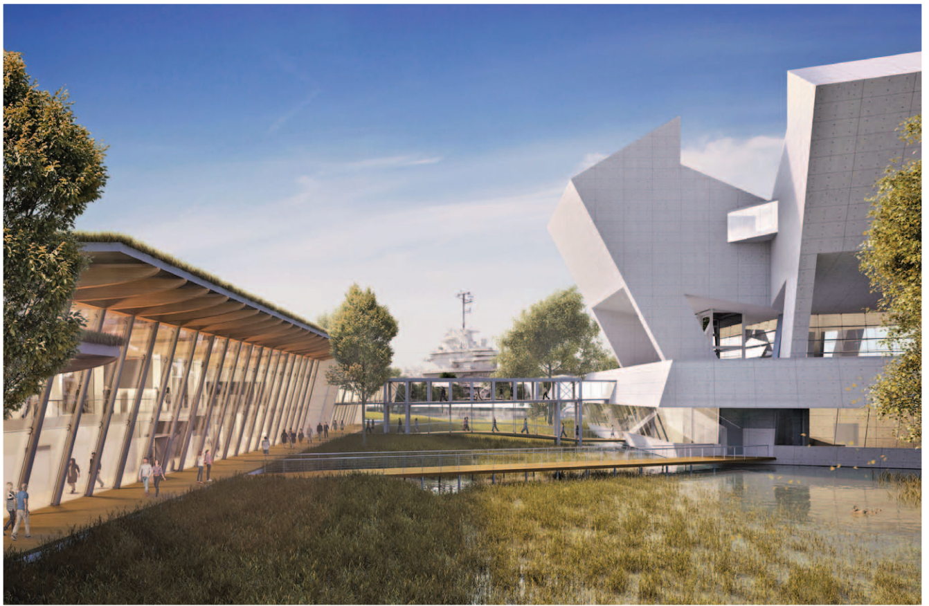
Construction on the three-building, 107,000-square-foot complex will begin in 2017 and take around 18 months to complete.
