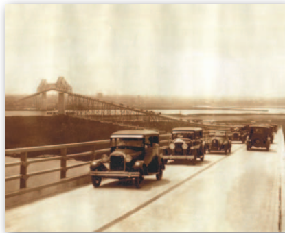
The John P. Grace Memorial Bridge was built at a cost of $6 million. Until 1945, there was a toll of 50 cents per vehicle and driver, with an additional 15-cent charge for each additional passenger.
